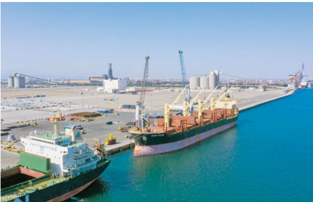
NEW FACILITY: The overall project will see the construction of 700m quay wall for an upcoming facility in the eastern area at Sohar Port. - File picture
