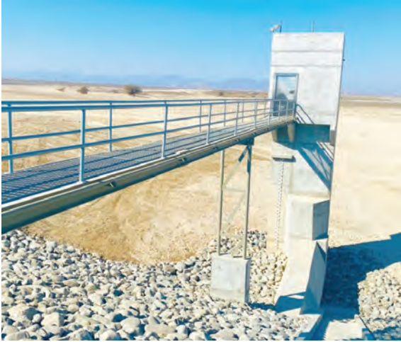
The works included repairing landslides, enhancing groundwater recharge efficiency
