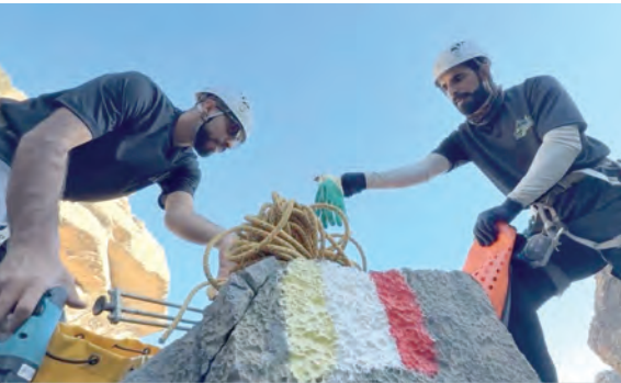
Works included replacing old supports with 48 stainless steel anchors.
