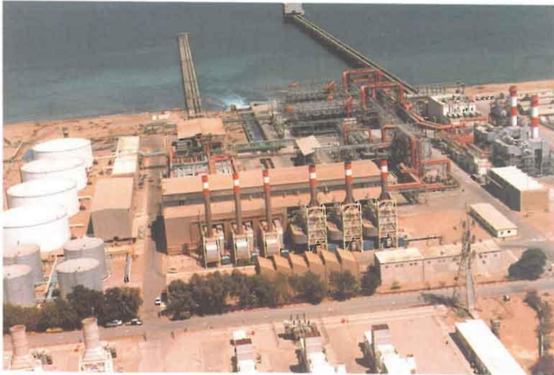
The extensive desalination installation at Ghubra which supplies much of the Muscat area's needs for electricity and water
