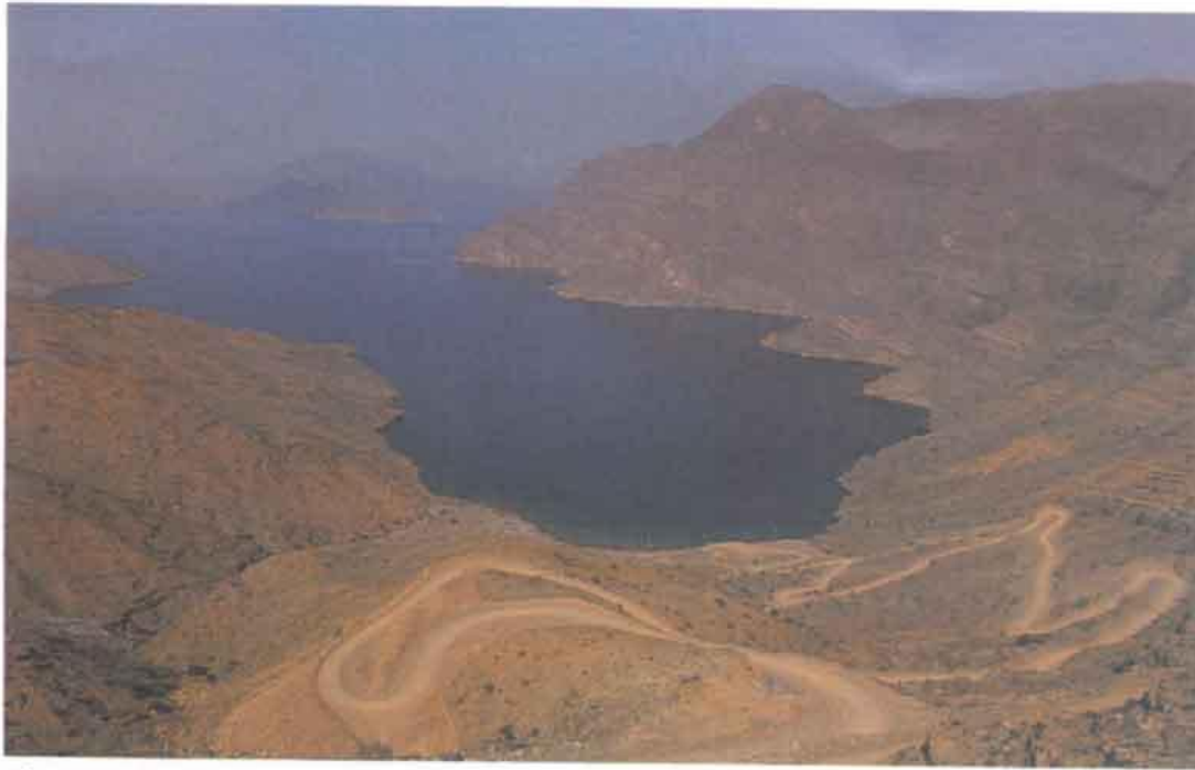
The majestic Jebel Musandam, commanding the vital Strait of Hormuz through which much of the world's oil supplies flow. The road in the foreground is an impressive testimony to the skill of engineers of the Sultan's Armed Forces
