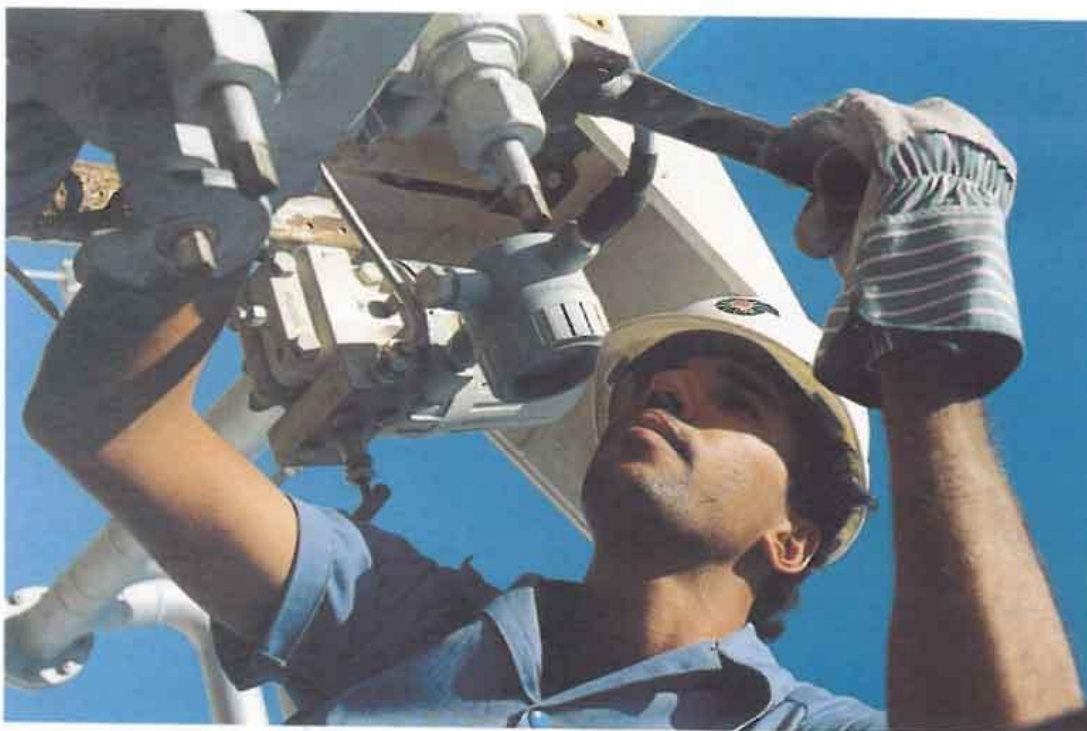
An oilfield technician carries out maintenance work on pipelines in the Interior (Photo: P.D.O.)
