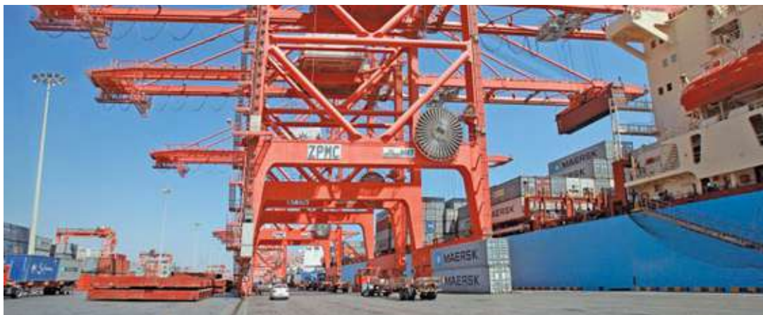
INVESTMENT OPPORTUNITIES: The facility will lend strong support to the logistics sector in the Sultanate, enhance the global supply lines with innovative solutions and open up investment opportunities for national and foreign industries.
