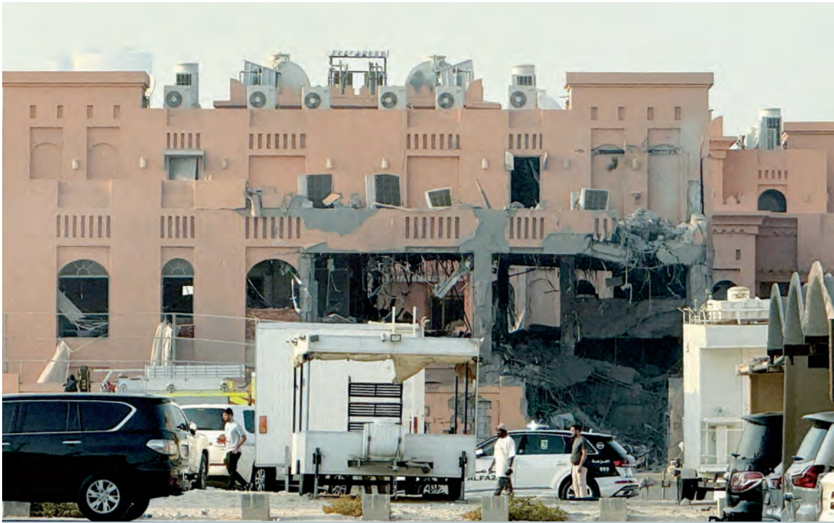
A damaged building following an Israeli attack on Doha, Qatar, on Tuesday. — Reuters
