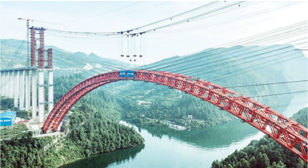
Wujiang grand bridge in SW China's Guizhou completes closure Aerial picture shows the construction site for the closure of Wujiang grand bridge, a main project of the expressway linking Dejiang and Yuqing, in southwest China's Guizhou Province. xinhua
