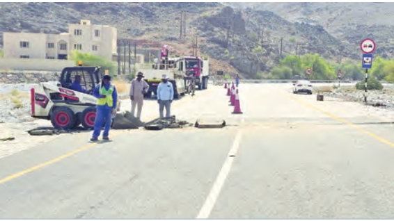
Repair work in progress on a road in Wadi Bani Kharous
