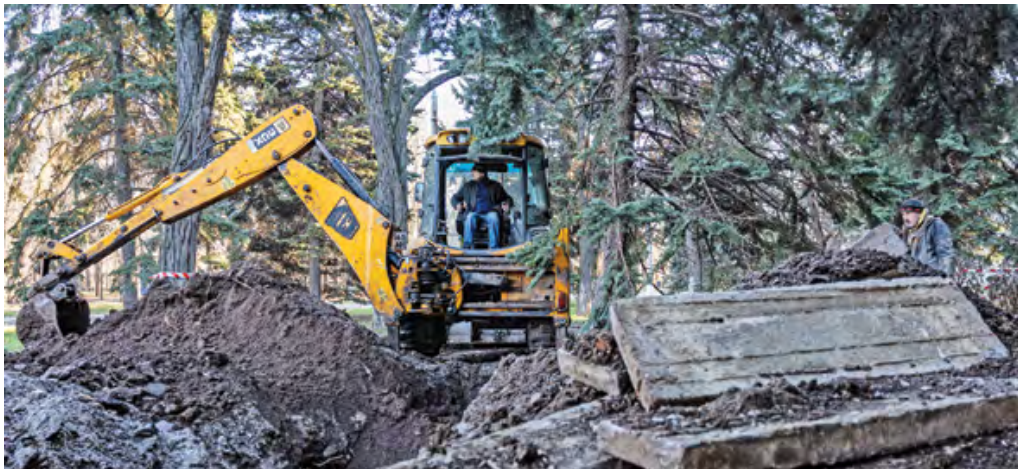
A technician mans an excavator as they repair heating pipes damaged during Russian shelling in the city of Kramatorsk, eastern Ukraine, on December 19 (AFP)
