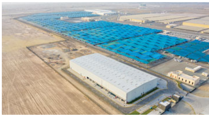
STRATEGIC PROJECT: Sohar Freezone is a 4,500-hectare project which has successfully leased 62 per cent of Phase 1 (as of 2020), with leasing now commencing for Phase 2. - Supplied picture
