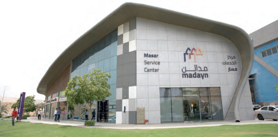
The phased plan includes around 90 strategic projects aimed at developing infrastructure and services in existing and new industrial cities.
