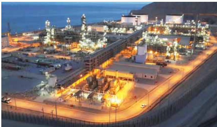
Musandam Power Plant co-located with the Musandam Gas Plant in the Wilayat of Bukha.
