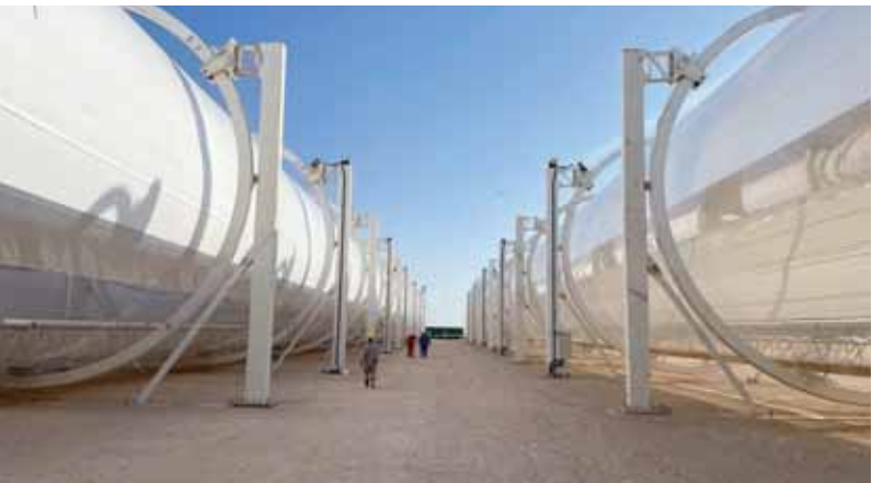
Inflatable tubes and mirror films at the heart of Heliomis' solar thermal powered water desalination plant set up at Qarat Al Milh (Credit: Heliomis)
