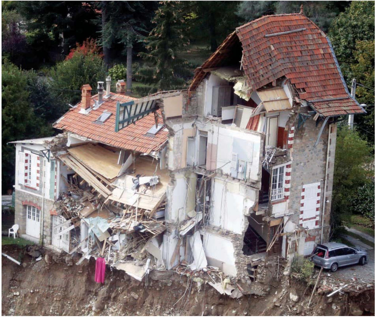
An aerial view shows damaged houses in Saint-Martin-Vesubie, southern France, as clean-up operations continue after storm Alex hit the Alpes-Maritimes department, bringing record rainfall in places and causing heavy flooding that swept away roads and damaged homes. — Reuters
