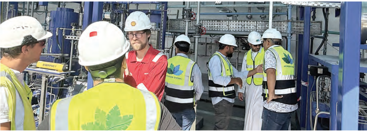
Representatives of Oman Shell and Saudi-contractor Hydrogen Systems pictured during a recent visit to the site of Oman’s first hydrogen refueling station under construction at Muscat International Airport (Picture credit: Hydrogen Systems)
