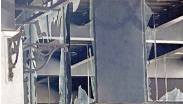
Windows at the Rameshwaram Cafe are seen broken after a low-intensity explosion which took place in Bengaluru on Friday (ANI)
