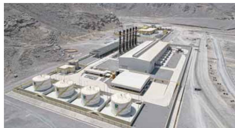
Power station in Musandam.
