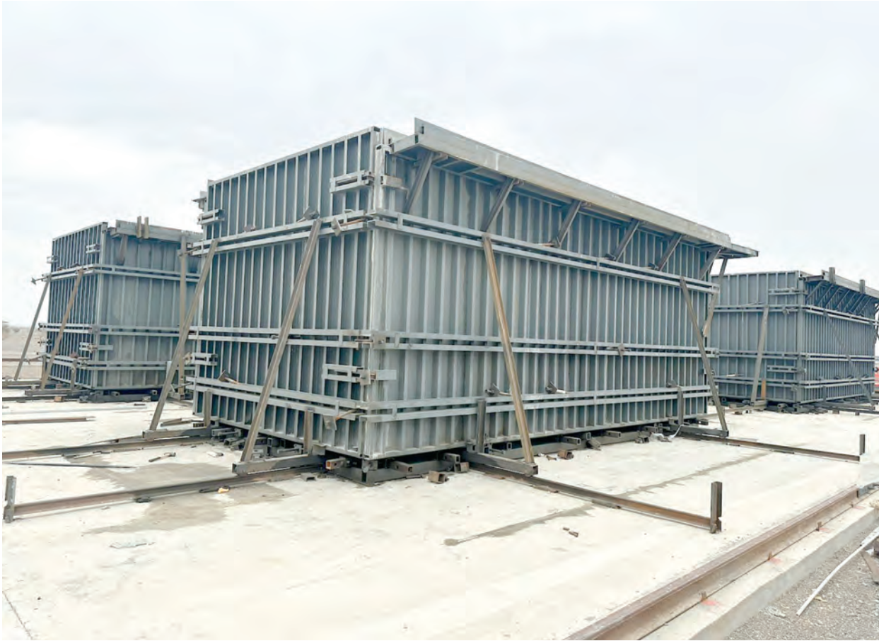
Construction underway of new projects at Al Mudhaibi Industrial City
