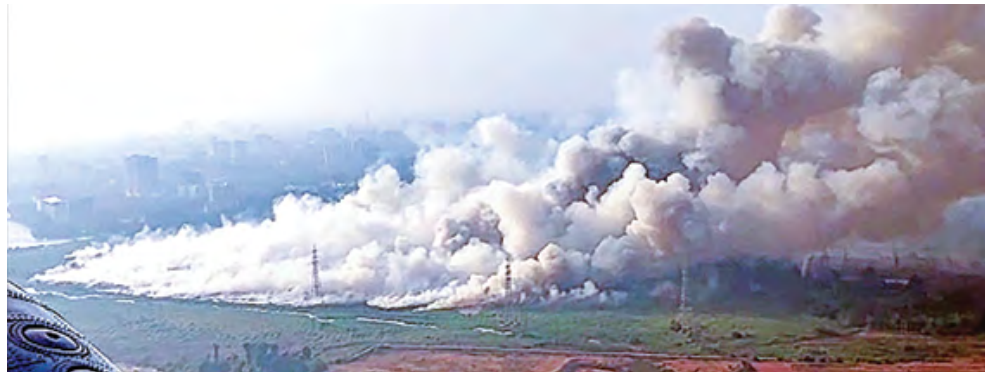
A massive fire broke out at the Brahmapuram waste plant in Kochi on March 2 (ANI)
