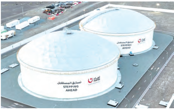
The system comprises 17 reservoirs with a combined storage capacity of 265,000 cubic metres, located in the wilayats of Al Qabil, Ibra and Al Mudhaibi.
