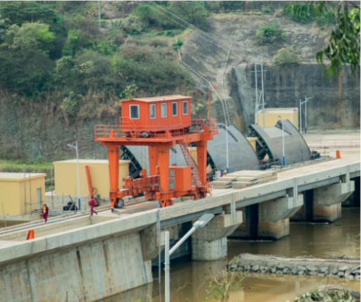
East Africa mega hydro power project nears completion Water flows through the open spillway gates upstream the waterfalls at the Rusumo border between Rwanda and Tanzania for the regional Rusumo Falls Hydroelectric Project. Construction of the regional Rusumo Falls Hydroelectric Project has reached an implementation status of 95 percent before operational, Nile Equatorial Lakes Subsidiary Action Program Coordination Unit (NELSAP-CU) said in a statement. Xinhua
