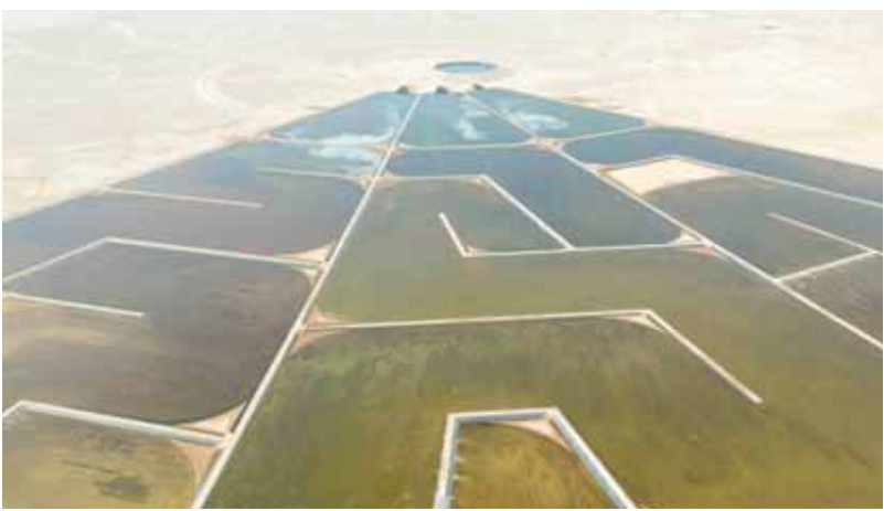
Rima Water Treatment Plant.
