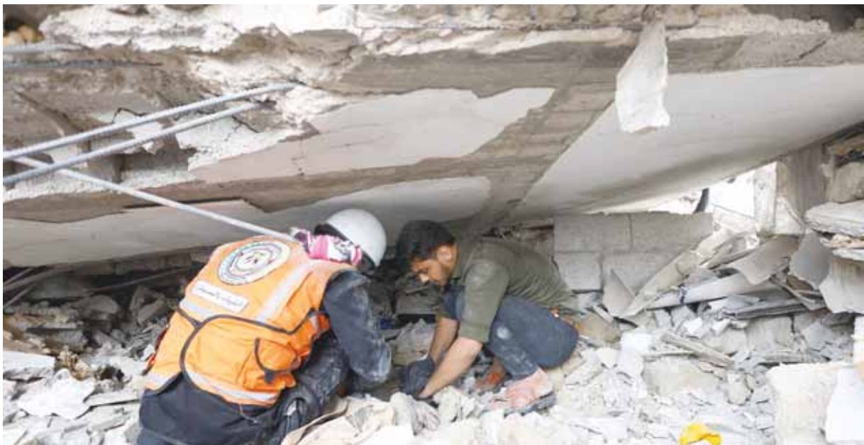
An Emergency worker and a Palestinian man check the damage at the site of Israeli strikes on houses, in Khan Yunis. — Reuters
