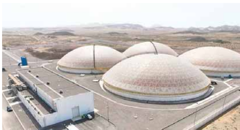
The water networks project aims to sustain water services in Liwa.
