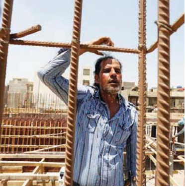
A worker cools himself while he works at a construction site during sweltering summer heat in Baghdad. — Reuters
