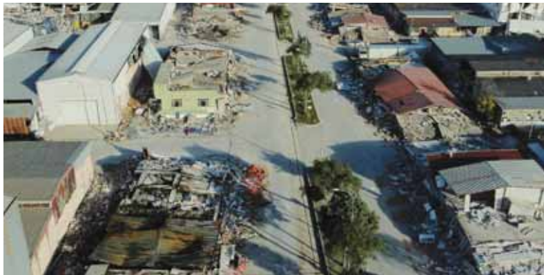
A general view of flattened buildings in Antakya Kucuk Sanyı Sitesi Industrial Estate is pictured in the aftermath of the deadly earthquake. - Reuters
