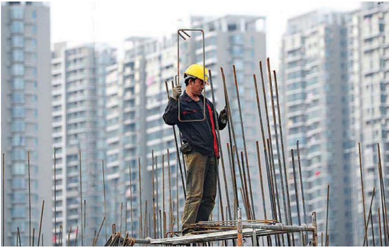
A man works at a construction site in central Beijing, China. — Reuters
