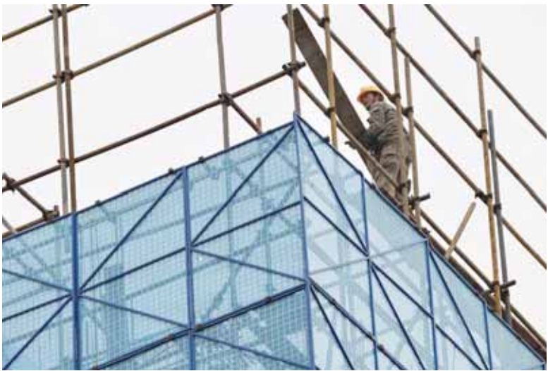
A man walks on a scaffolding at the construction site of the Beijing Xishan Palace apartment complex developed by Kaisa Group Holdings Ltd in Beijing. — Reuters
