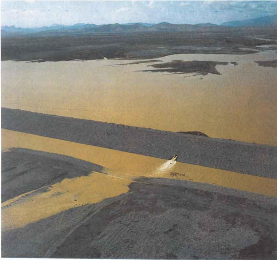
Water conservation is vital to the Sultanate: one of the recently constructed dams near Seeb (Photograph: CCEWR)
