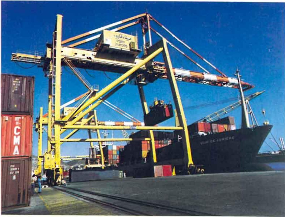
A ship discharges containers at Port Qaboos (Photograph: Port Services Corporation)
