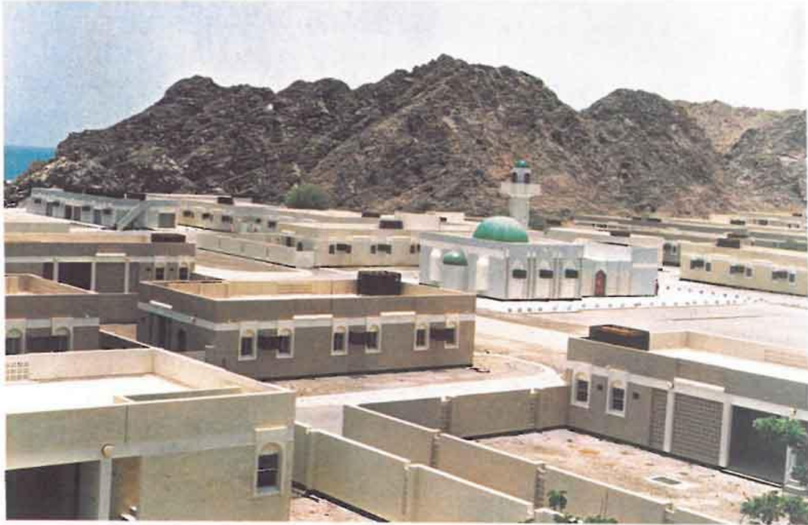
A Government-sponsored housing estate (Photograph: Ministry of Housing)
