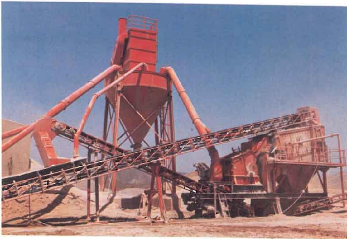
Dust control equipment operating at the Sohar Copper Mines. These air pollution control units are employed at industrial sites to avoid the danger of dust pollution of the atmosphere. (Photograph: Ministry of Environment and Water Resources)
