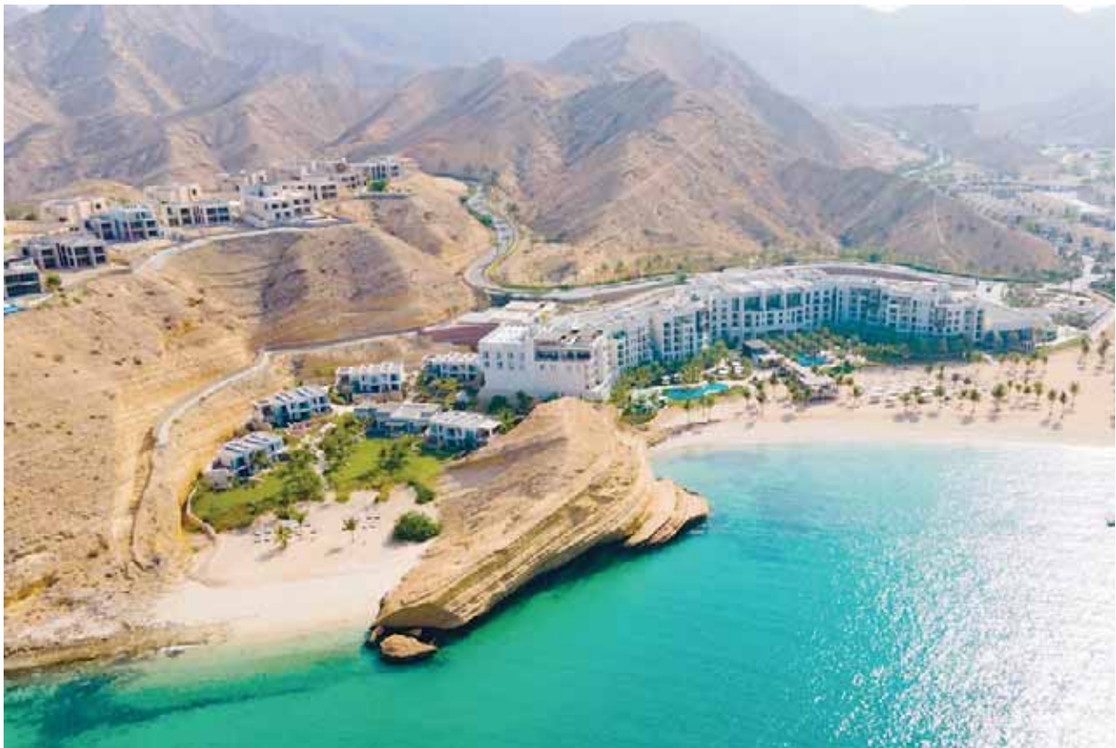
A general view of a 5-star hotel in Oman.
