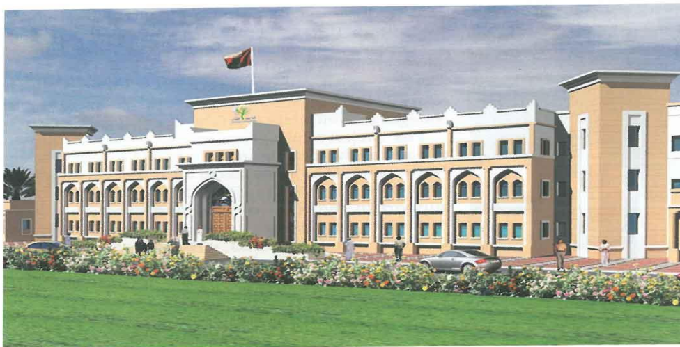
The government supports the private universities and colleges. Here Dhofar University, now under construction.
