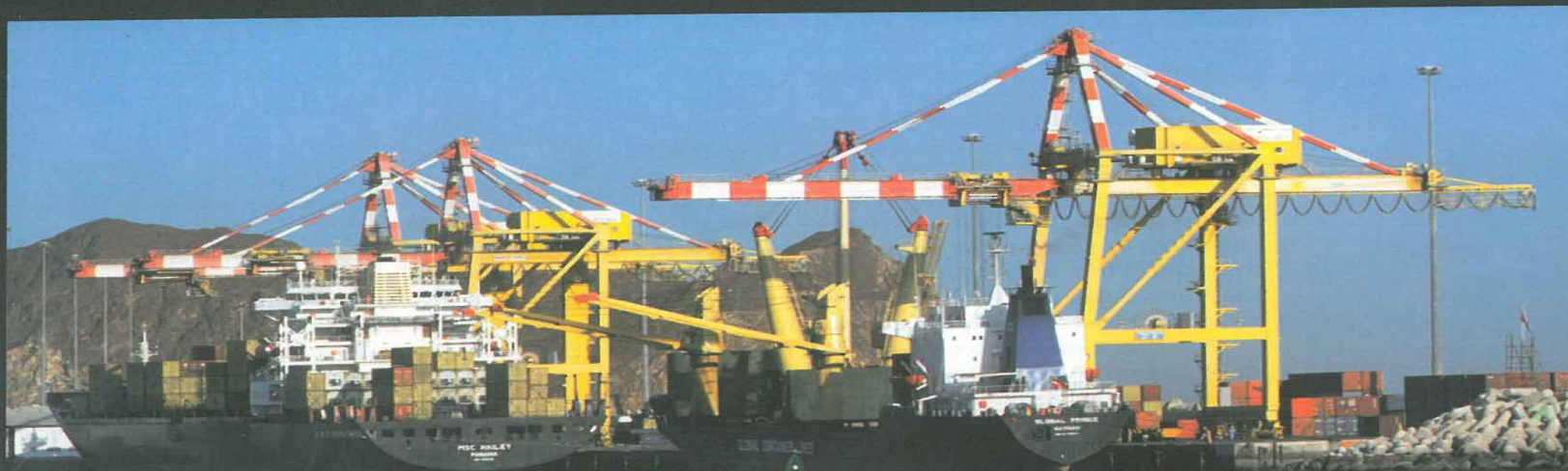
Port Sultan Qaboos in Muttrah - developing and expanding, particularly in the range of services it provides.
