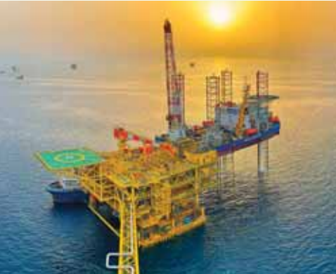
Setting Global Benchmarks: Hasbah-II Offshore Project, KSA
