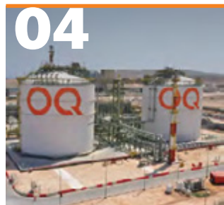
OQ's $463mn ammonia plant begins production
