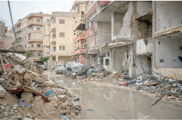
Destruction caused by Israeli shelling in the southern Lebanese city of Tyre.
