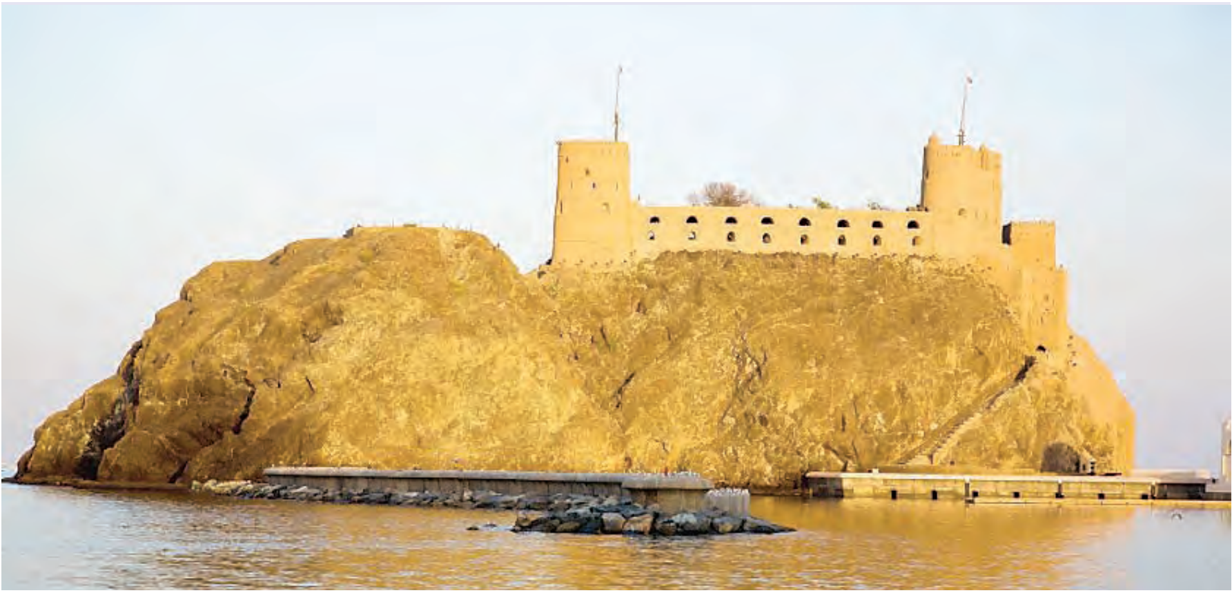
Al Jalali Fort lies on a rocky outcrop on the east side of the Muscat harbour.
