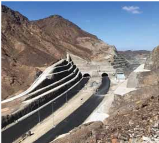
FIRST TUNNELLED ROAD OPENS IN OMAN
