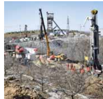
Members of a rescue team work at the site of a gold mine explosion where 22 miners are trapped underground in Qixia, in eastern China's Shandong province. — AFP
