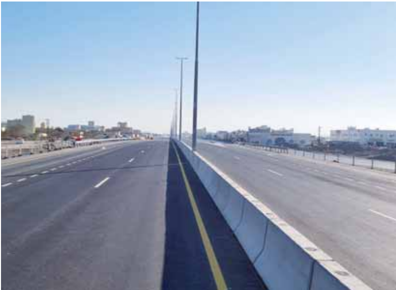
lanes in each side, (2.5m wide) external asphalt road shoulders, and (1.5m wide) internal asphalt road shoulders. — ONA
