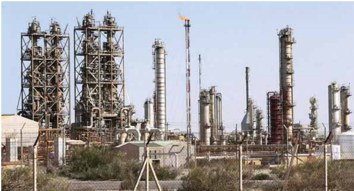
Pipelines are seen at the oil port of Brega, Libya, in this file photo. – Reuters
