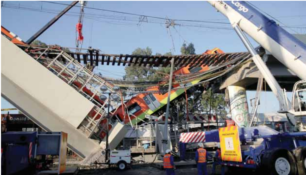
Cranes work at a site where an overpass for a metro partially collapsed with train cars on it at Olivos station in Mexico City, Mexico on Tuesday. — Reuters
