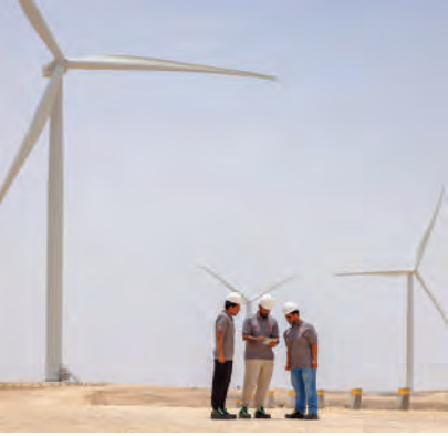
Dhofar wind power project in Harweel
