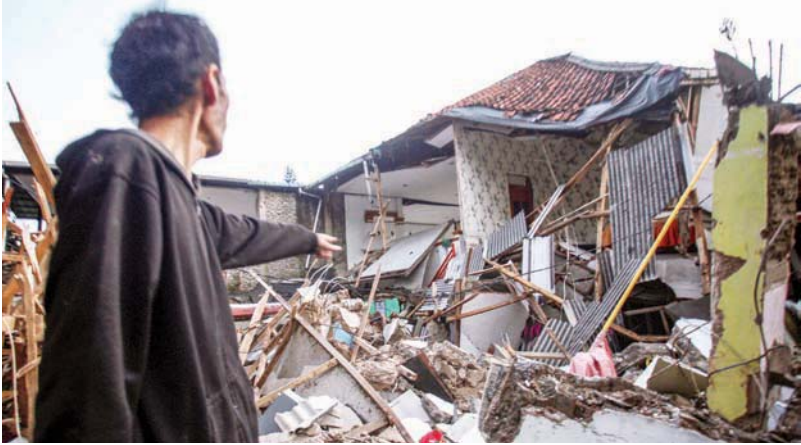
A local stands near houses damaged after earthquake hit in Cianjur, West Java province, Indonesia, on Monday. — Reuters
