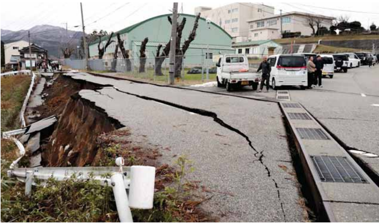
People stand next to large cracks in the pavement after evacuating into a street in the city of Wajima, Ishikawa prefecture. – AFP
