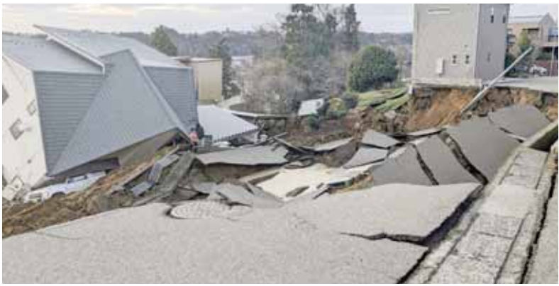
A view of a collapsed road and houses because of an earthquake in Wajima, Ishikawa prefecture on Monday. - Reuters
