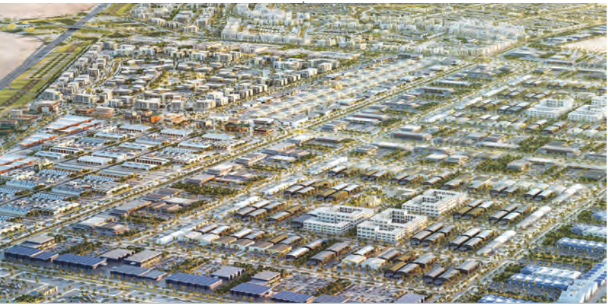
The development currently supports over 33 industrial and logistics projects under construction, spanning across six key economic sectors.
