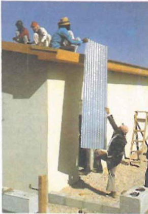
Low cost housing is provided by the government
