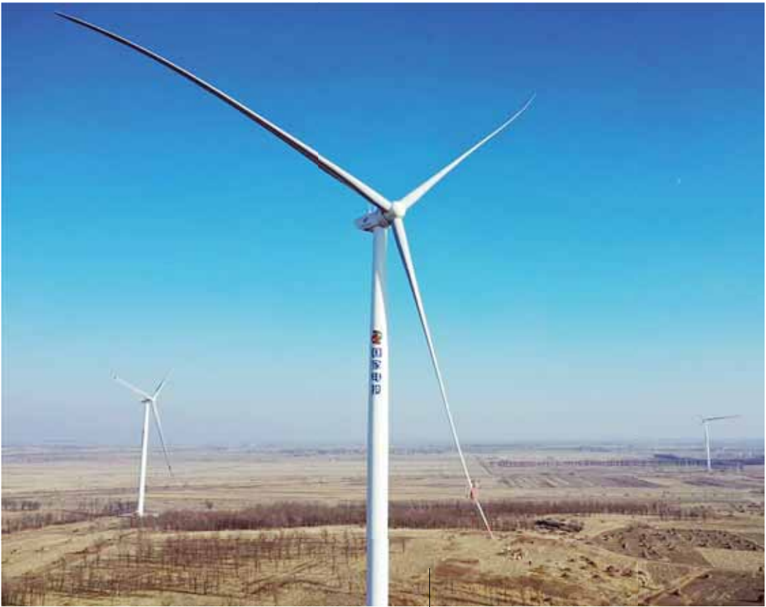
Major wind power project goes into operation in NE China The picture shows a major onshore wind power project in northeast China's Liaoning Province. Liaoning Province in northeast China saw a major onshore wind power project connect to the state grid and became operational on Saturday. xinhua
