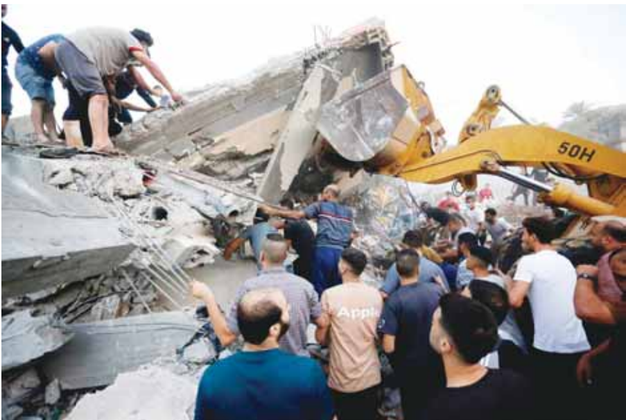
A bulldozer shifts the rubble of a building destroyed following an Israeli attack on the town of Deir Al-Balah, in the central Gaza Strip. – AFP
