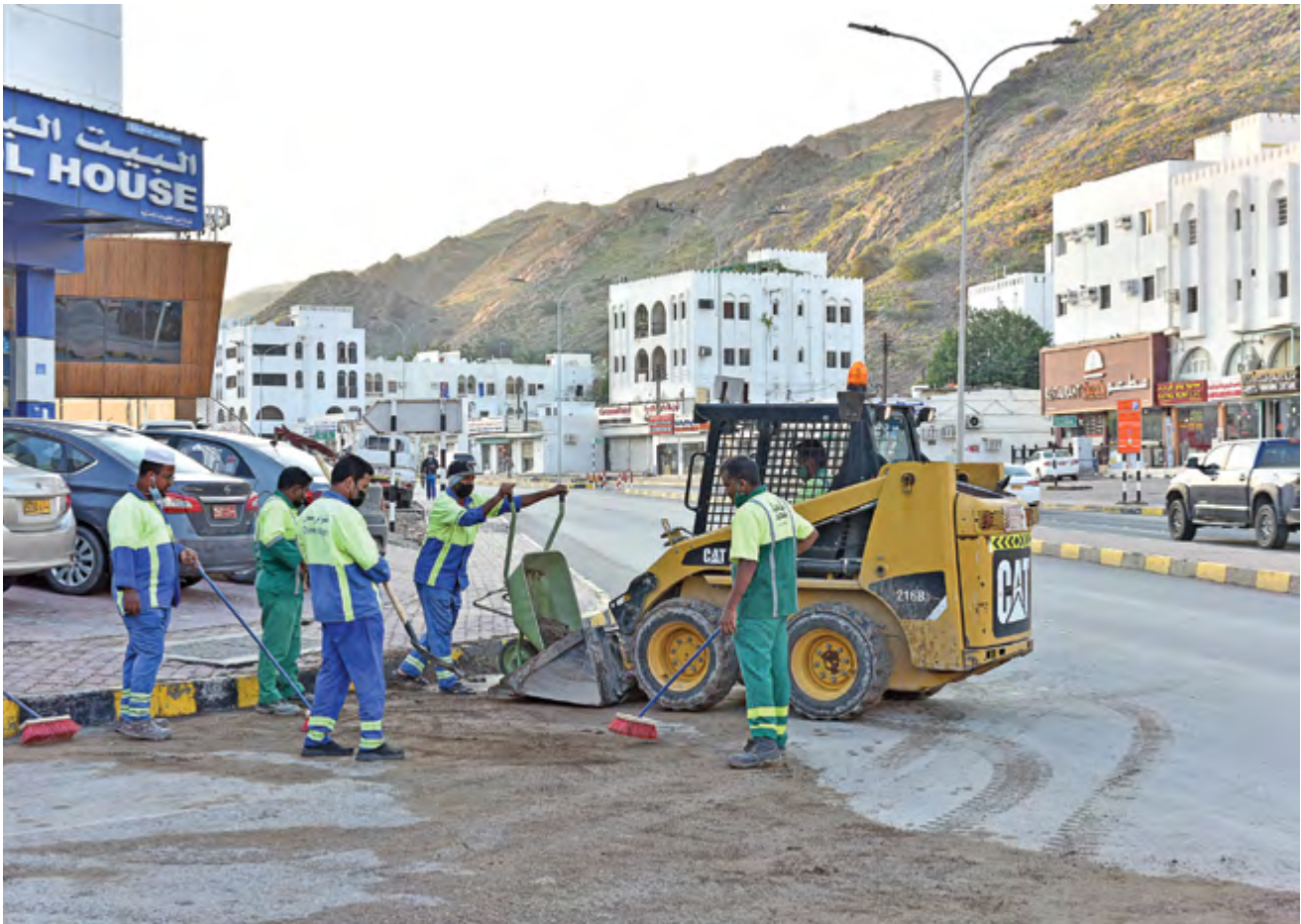
Muscat Municipality deployed teams for much needed clean-up and road repair works across the city on Wednesday following the heavy rains that affected several parts of the sultanate caused by a low-pressure system named Al Azm on Tuesday (Muscat Daily)
