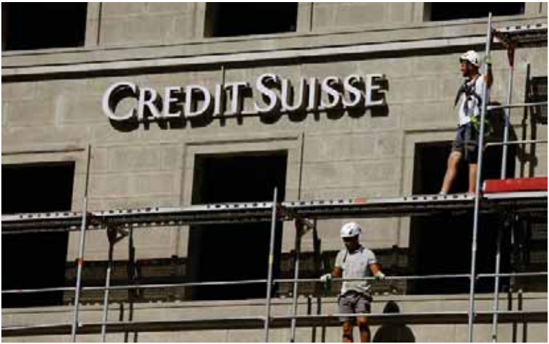
Workers are seen in scaffolding in front of Credit Suisse building in Zurich. – AFP
