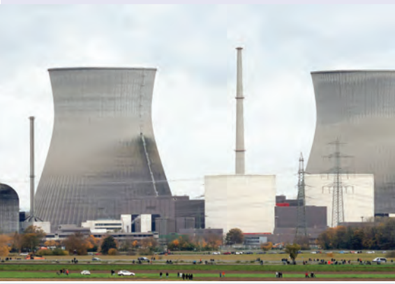
The decommissioned nuclear power plant Gundremmingen in Gundremmingen, southern Germany, prior to the controlled demolition of the plant's two cooling towers and after the controlled demolition. — AFP
