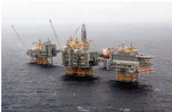
An aerial view shows five platforms over the Johan Sverdrup oil field in the North Sea, some 140km west of the town of Stavanger, Norway (AFP)
