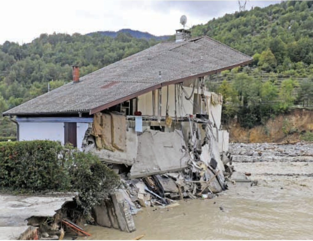
A house destroyed by the floods of the Vesubie river in Roquebilliere, southeastern France, on Saturday (AFP)
