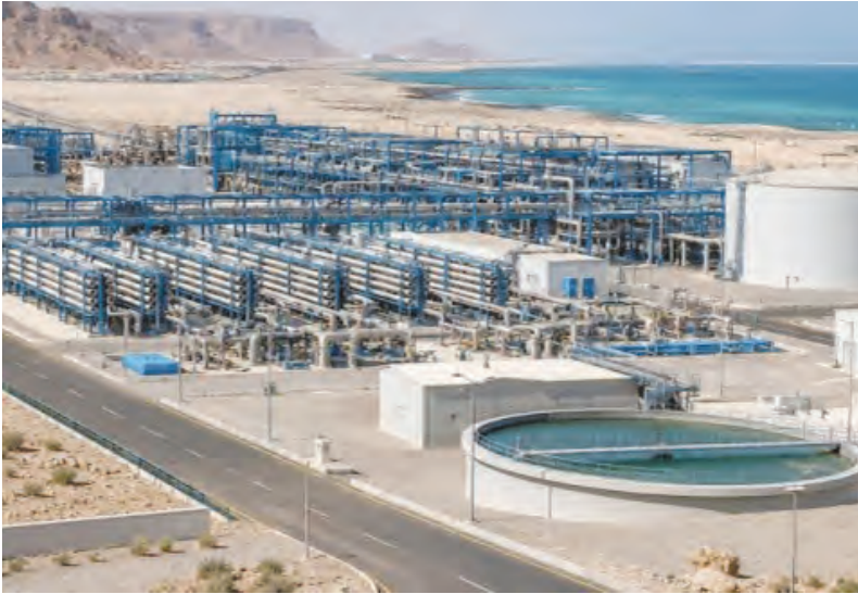
The plant will produce industrial water to support Meranti's upcoming direct reduced iron (DRI) and hot briquetted iron (HBI) plant at Al Duqm
