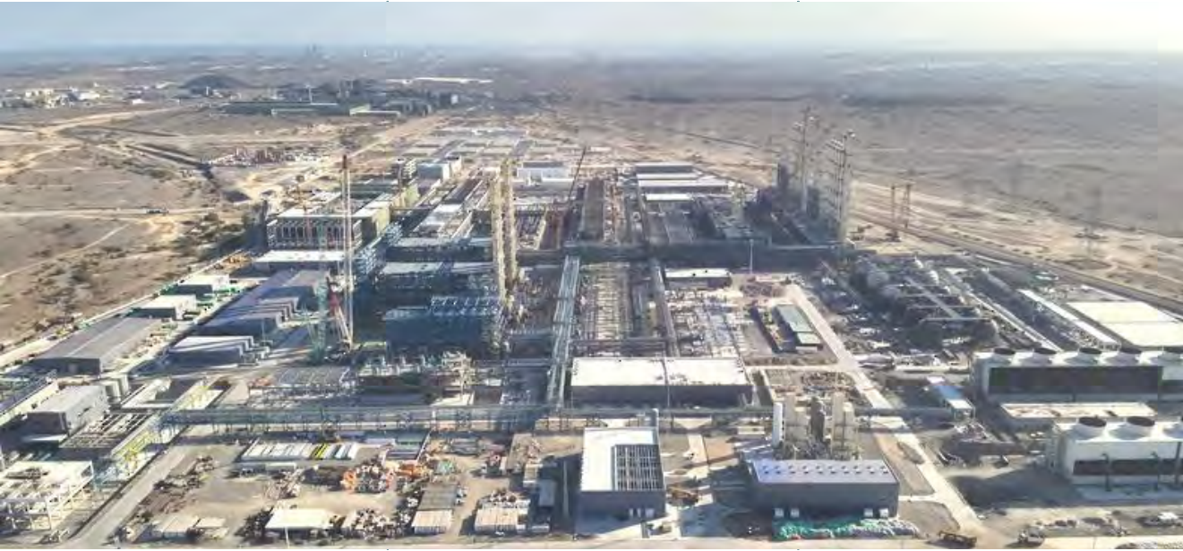
The polysilicon plant of UPS is set to be the largest project by power demand size to be connected to the grid this year.
